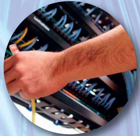
Cabling Plants Rehabilitation
