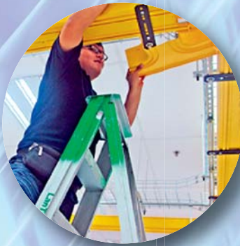
Cable Containment Installation (M&E) (Ladder, Basket, Tray, Trunking, Mat, etc)
